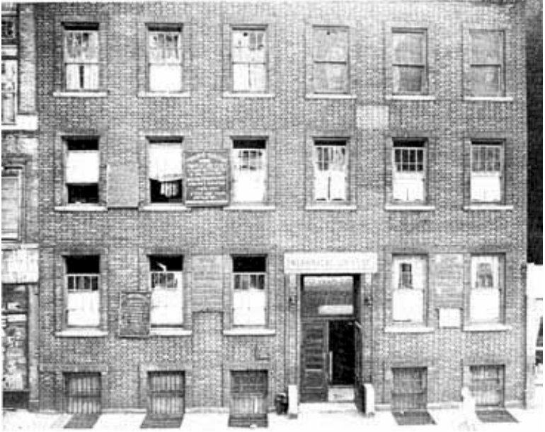
Building at 9-11 Montgomery Street (1915-21)
